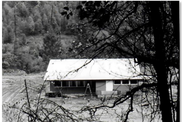
The New Denny School renamed "Grover Ladd", under construction
